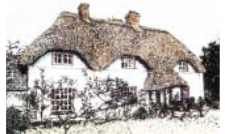
SUMMERHAUGH COTTAGE One of the buildings forming a prominent group around the old village square, along with The George Inn and Fourways.
