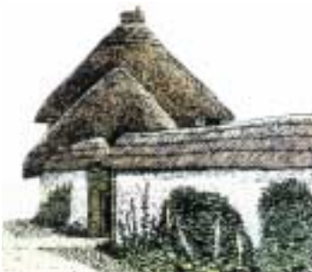
THE LODGE OR ROUNDHOUSE AND THATCHED COB WALL This unusually shaped building was built as a lodge for Stoke house – the remains of the long drive can still be traced by the side of the house. The thatched, chalk cob wall which dates from around 1800 A.D. is becoming a rare feature as the thatch is replaced by tiles.
